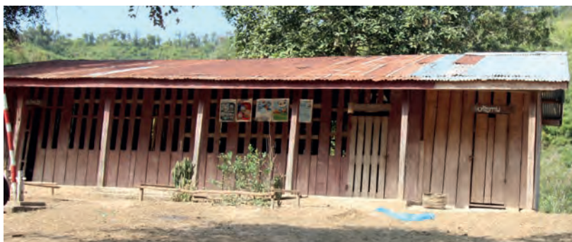
Houay Loa School, Laos before rebuilding
